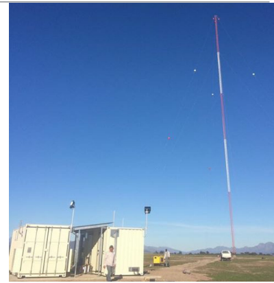
Picture: The completed facility as installed for Magic 828, in the Western Cape
